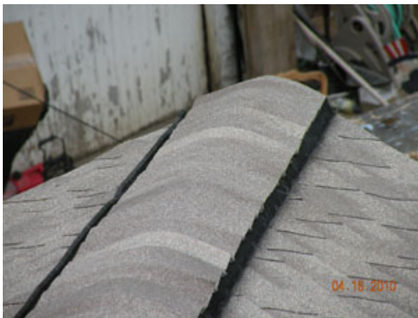
Hip Ridge Vent shingled-over.
